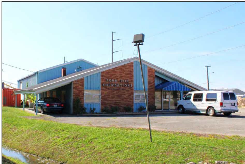
View of Commercial Building/Office (VDHR# 134-5323) Looking West
