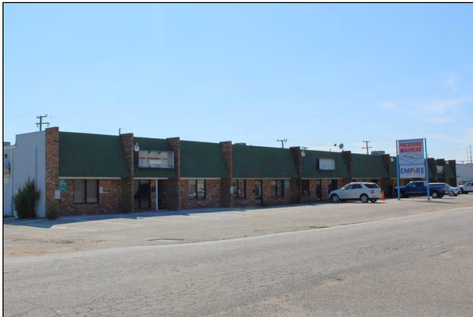
View of Commercial Building (VDHR# 134-6129) Looking Southwest
