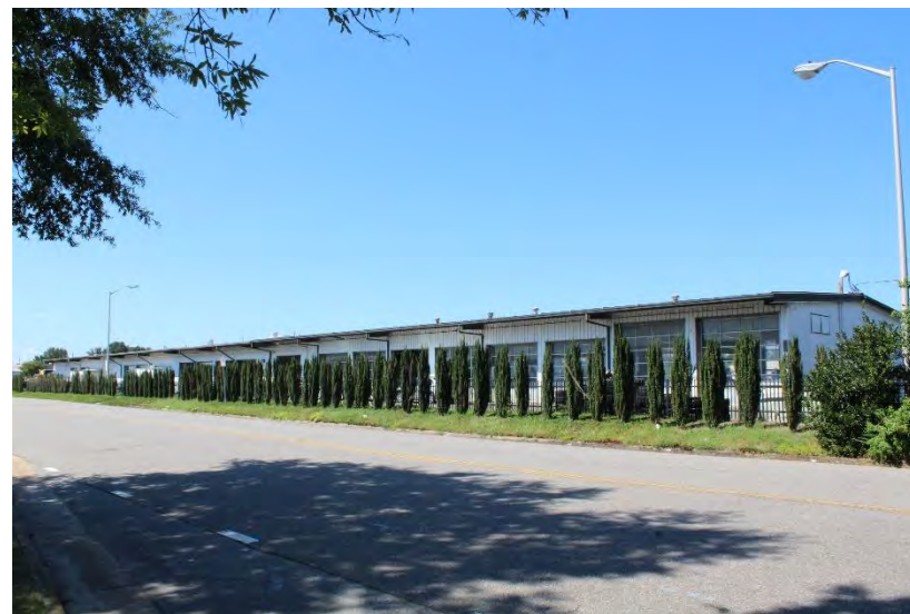
View of 1970 Service Garage looking northwest
