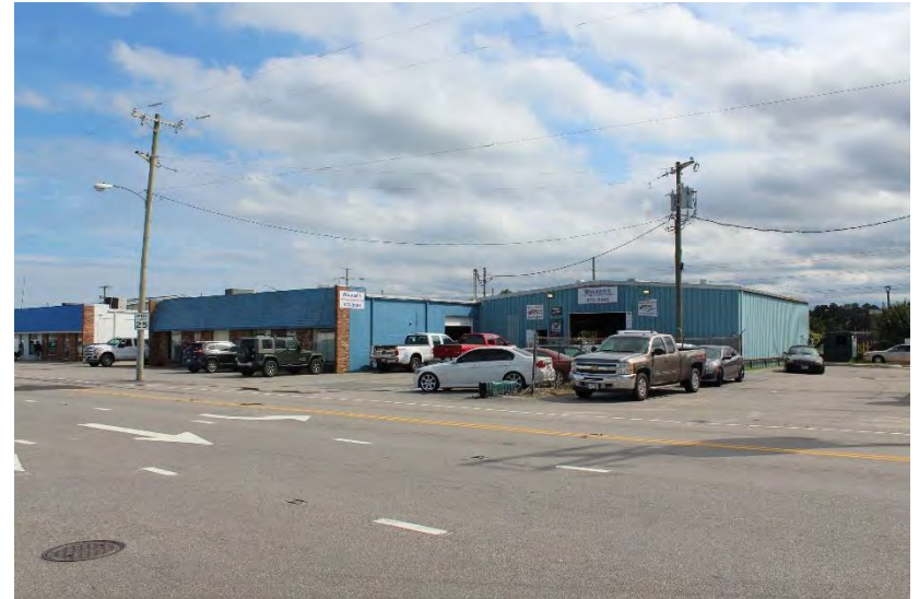
View of 5047-5049 and 5053 (warehouse) Cleveland Street looking southeast
