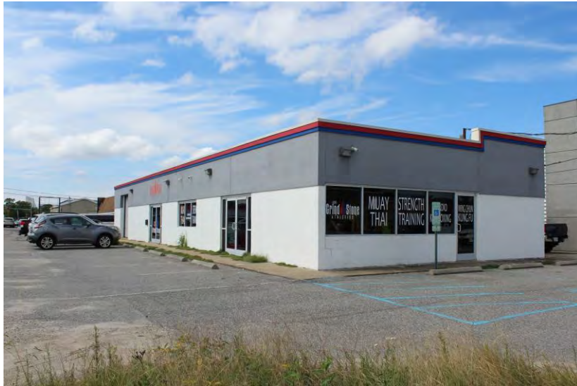
View of building looking northwest
