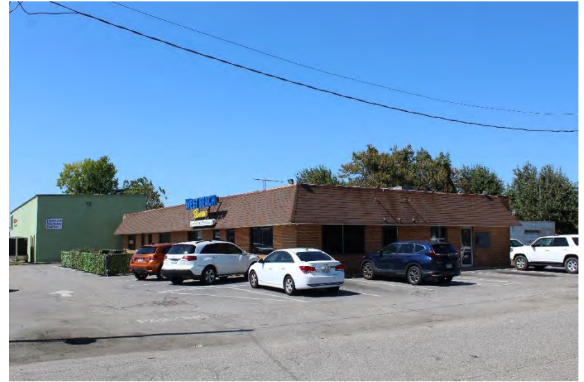
View of building looking northwest
