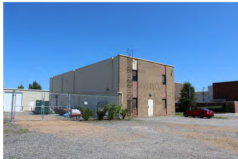
View of building looking southwest
