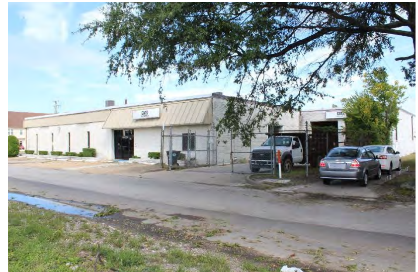
View of building looking northeast
