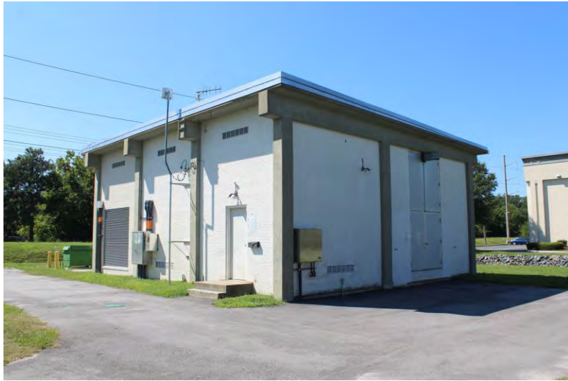
View of building looking southwest
