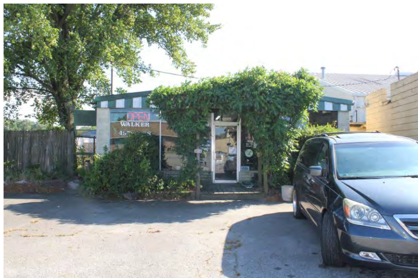
View of building looking south
