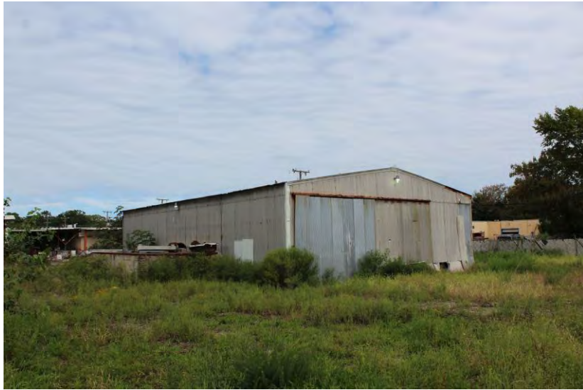
View of warehouse looking northeast
