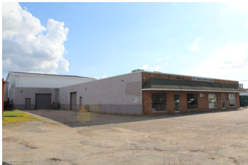
View of building looking southwest
