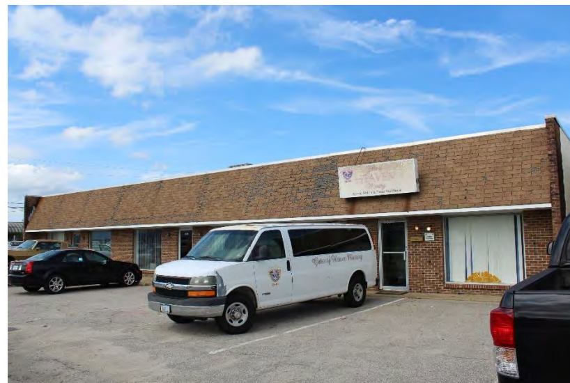
View of building looking northwest
