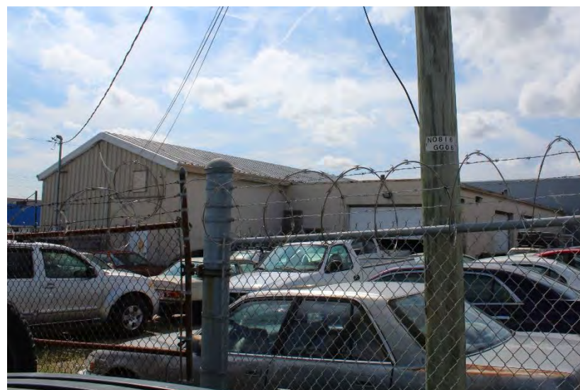
View of building looking southwest
