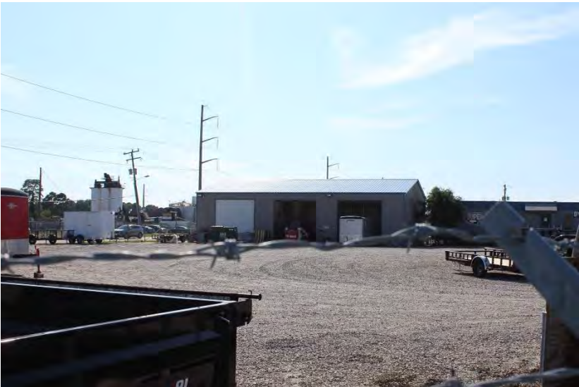
View of office and garage looking east
