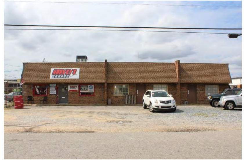
View of building looking west
