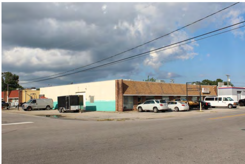
View of building looking northeast
