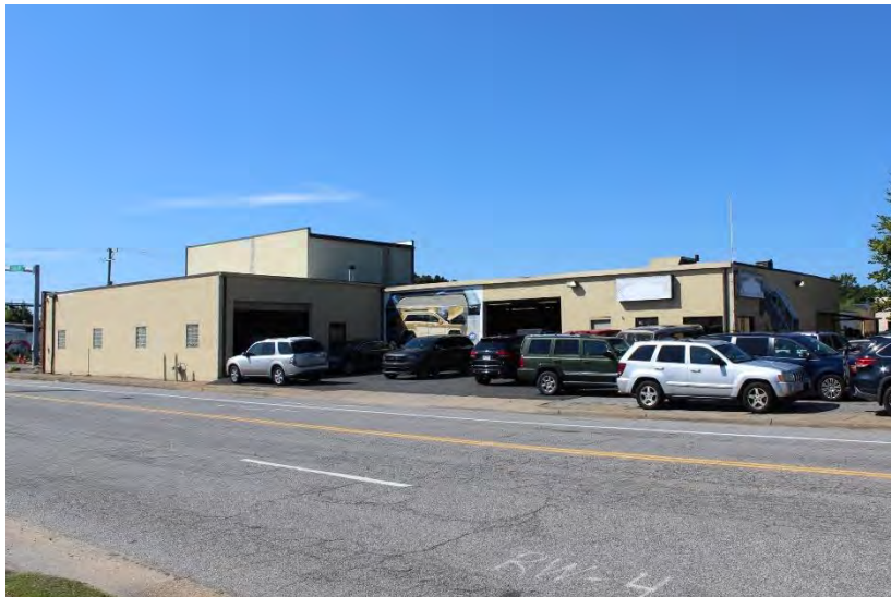
View of building looking northwest
