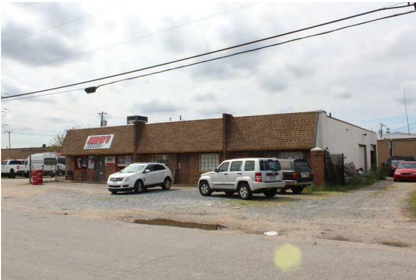
View of building looking southwest
