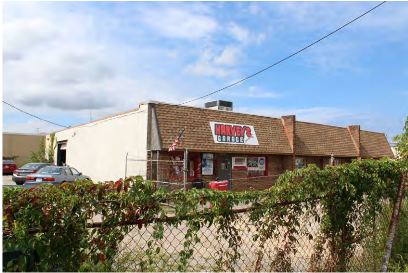
View of building looking northwest
