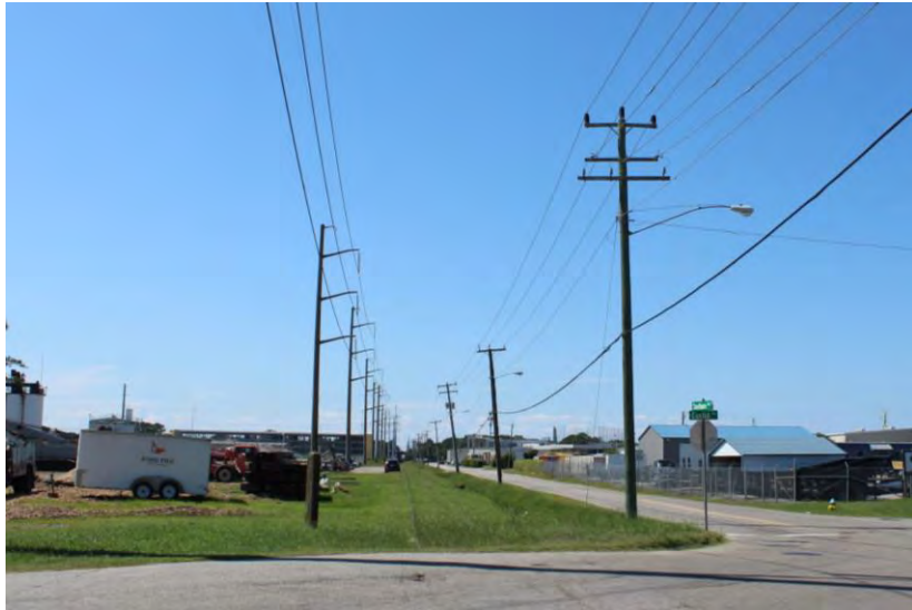
View of railroad bed looking west from Euclid Road
