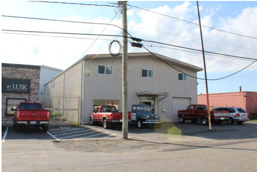
View of building looking northwest
