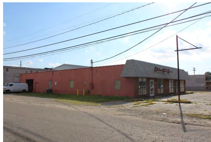
View of building looking southwest
