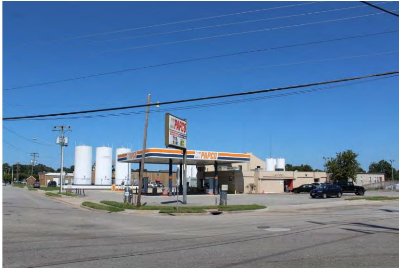
View of Papco property showing 1990 storage silos, gas station canopy, and office building, looking northeast
