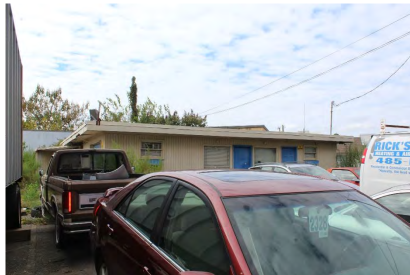
View of building looking southwest
