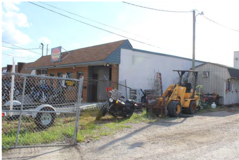
View of building looking southwest
