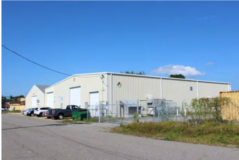
View of industrial building looking northeast
