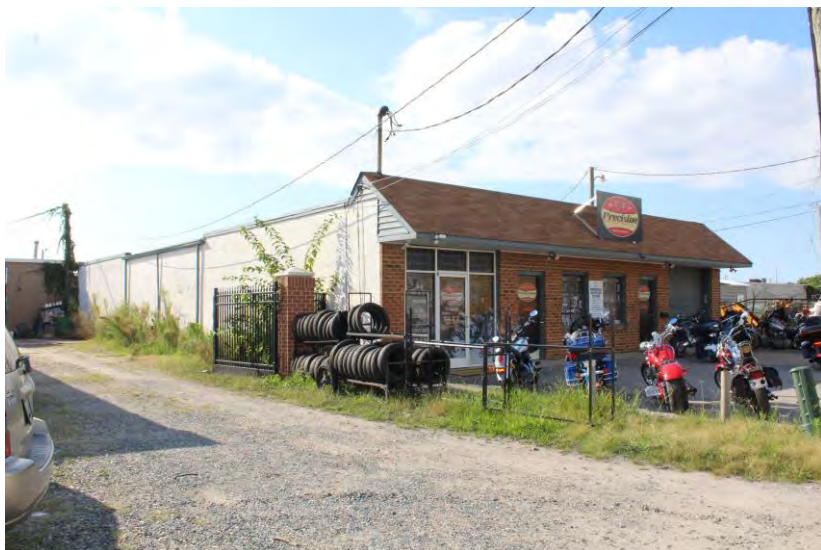
View of building looking northwest
