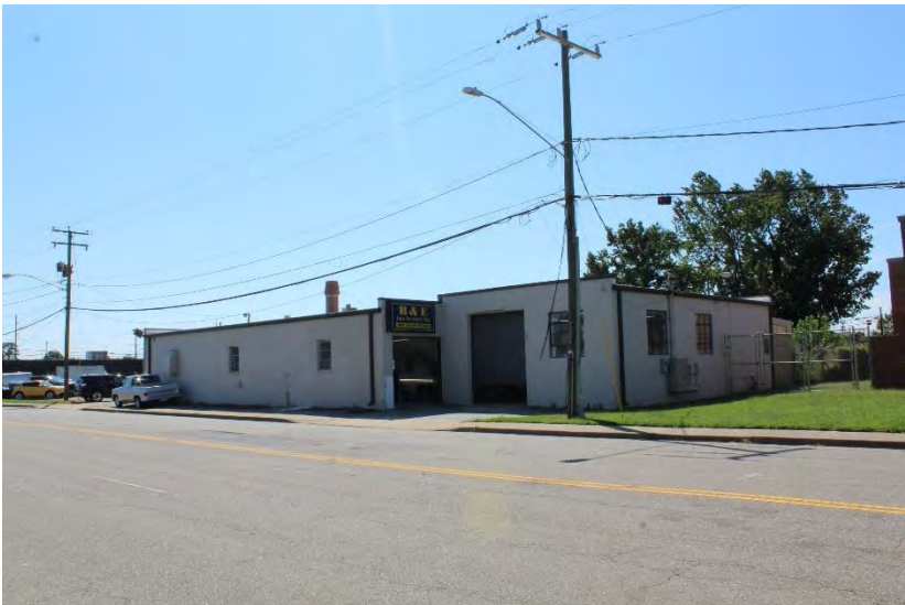
View of building looking southwest
