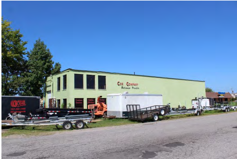
View of building looking northeast
