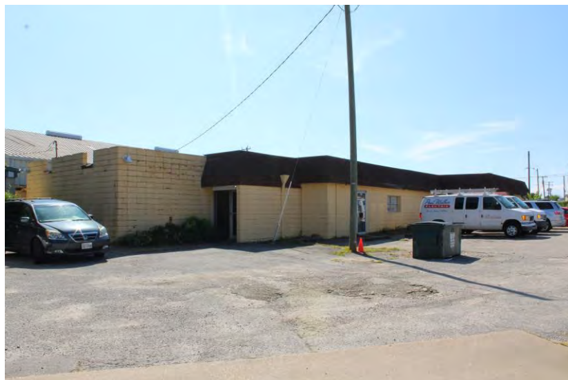
View of building looking southwest
