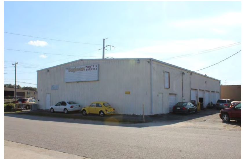
View of building looking southwest
