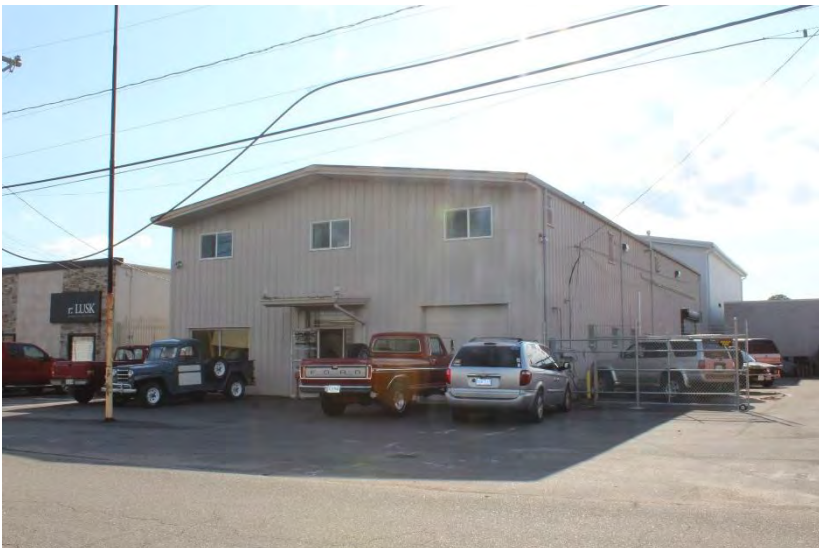
View of building looking southwest
