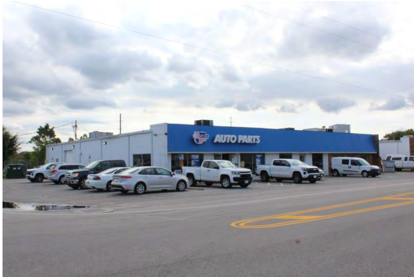
View of 5041-5045 Cleveland Street looking southwest
