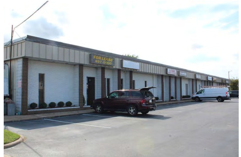
View of building looking southwest
