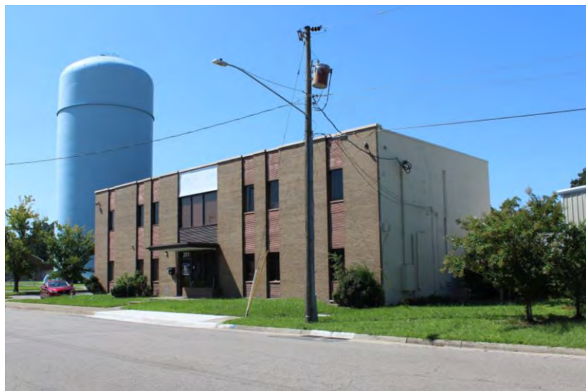
View of building looking southwest
