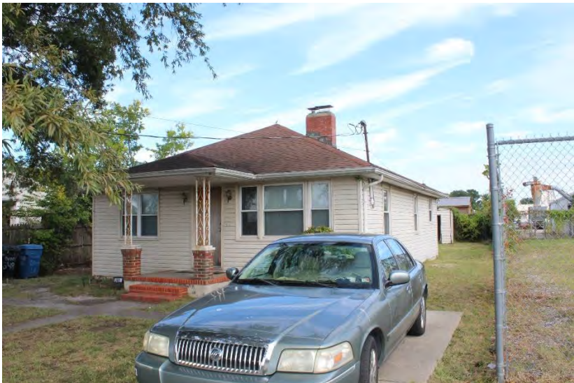
View of house looking northeast
