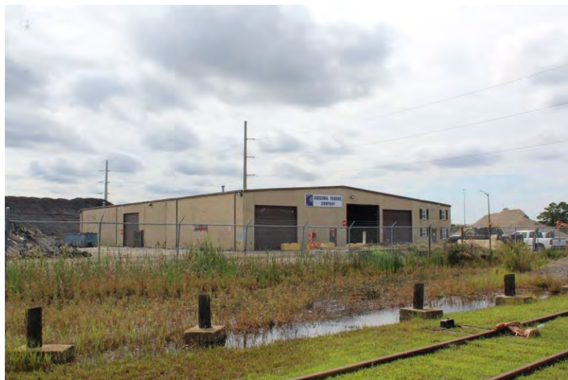
View of building looking southwest
