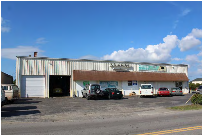
View of building looking northeast
