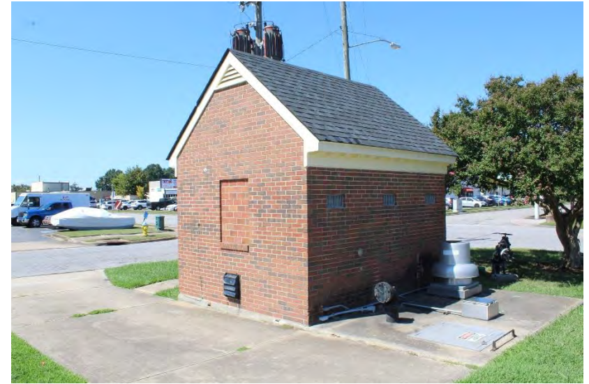
View of building looking northwest
