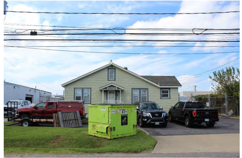
View of office looking west
