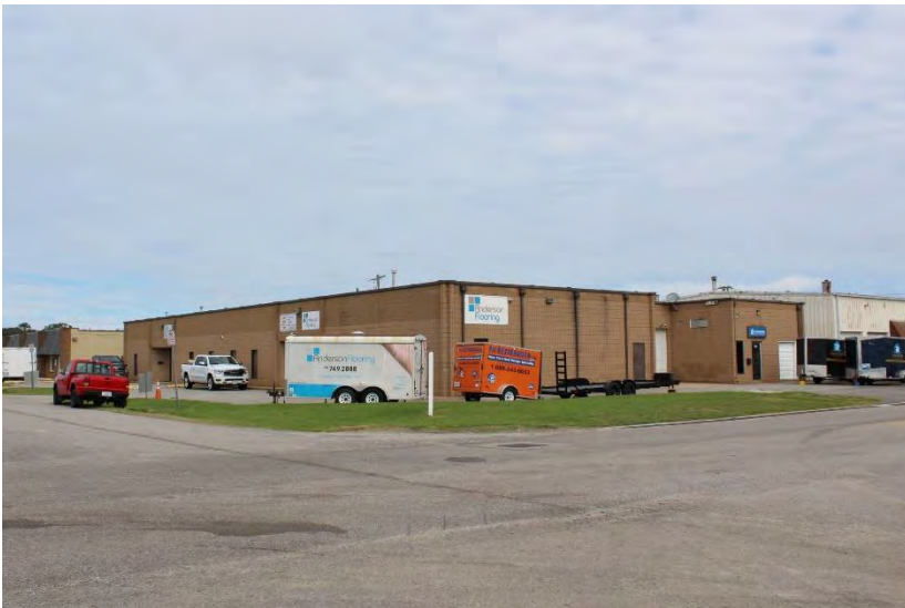
View of building looking northeast
