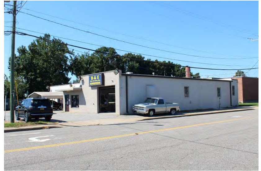
View of building looking northwest
