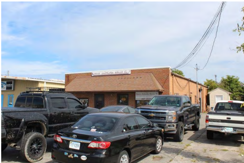
View of building looking northeast
