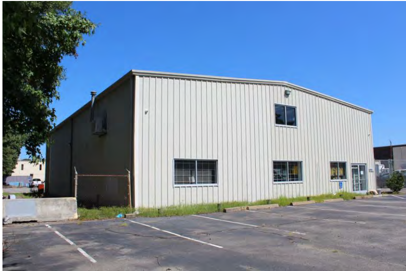
View of warehouse looking northeast
