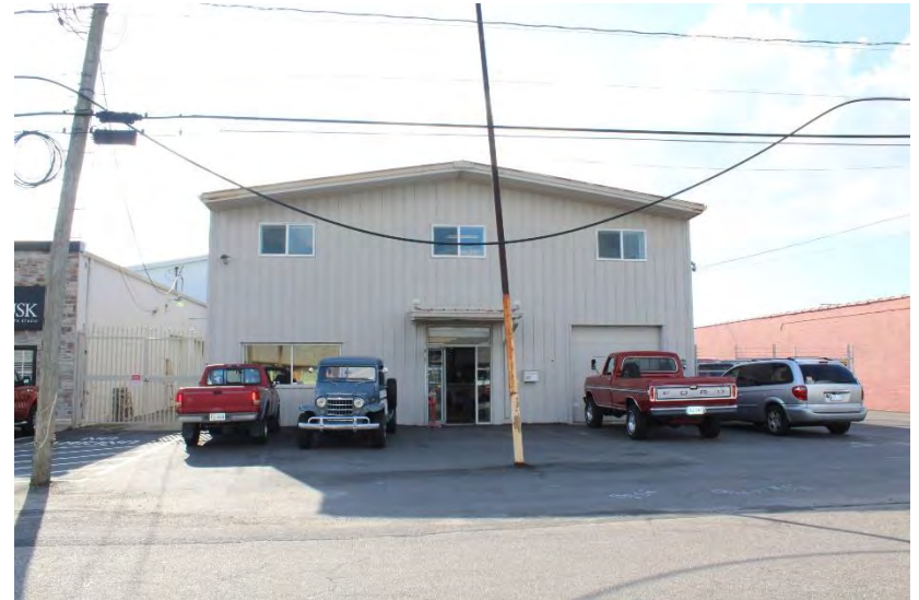
View of building looking west
