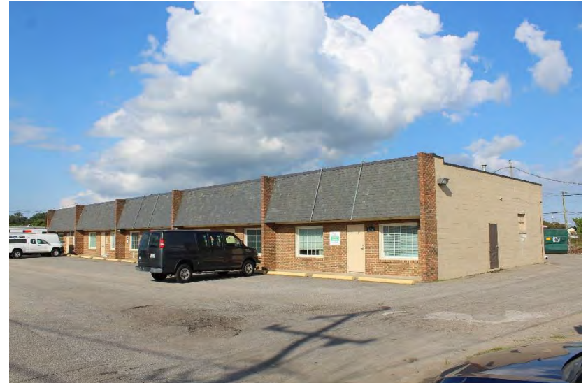
View of building looking northeast
