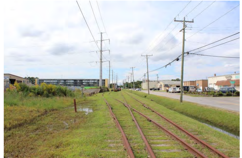
View of railroad segment between Dorset Avenue and Mac Street, looking west
