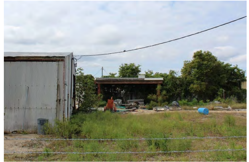
View of shed looking west
