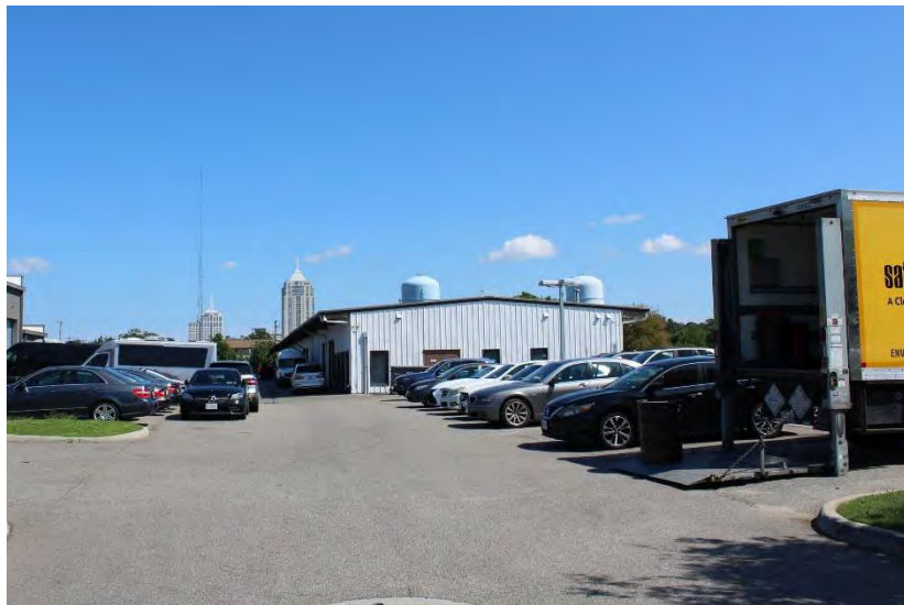
View of 1970 Service Garage looking east
