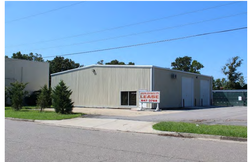
View of warehouse looking southwest
