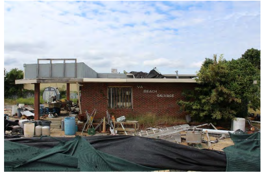
View of building looking west
