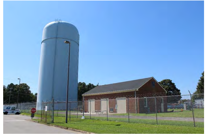
View of south water tower and utility building looking southwest
