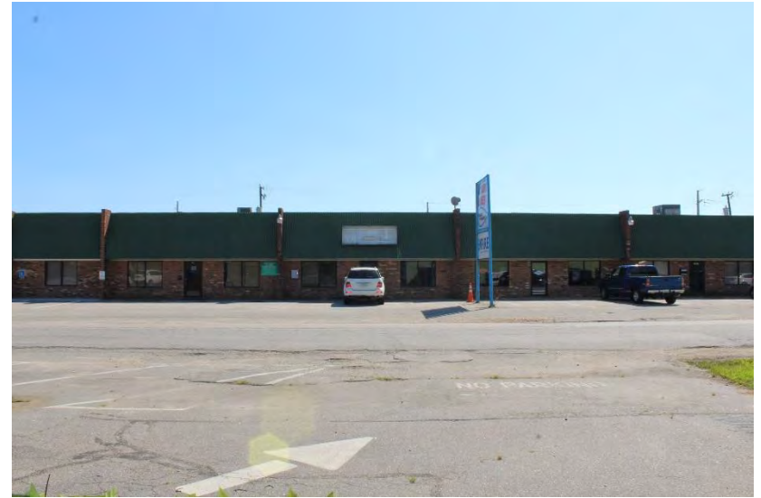
View of building looking south
