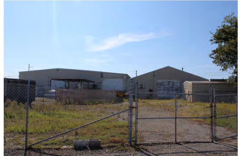
View of industrial building looking west
