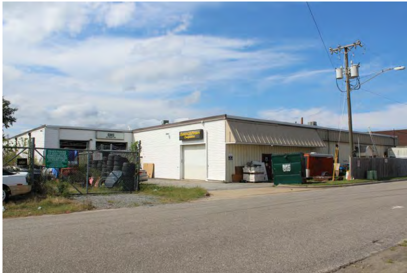
View of building looking northwest
