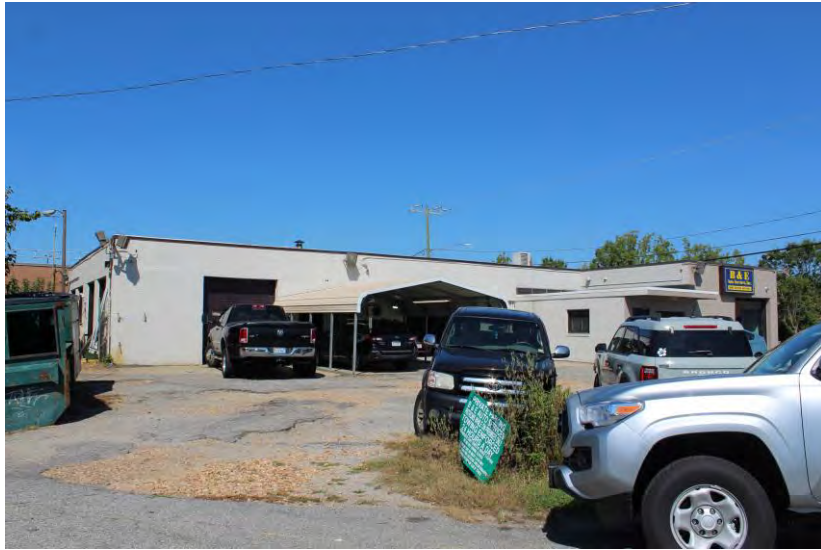
View of building looking northeast
