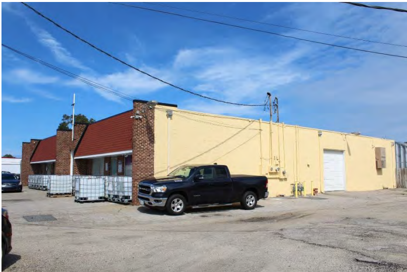
View of building looking northeast
