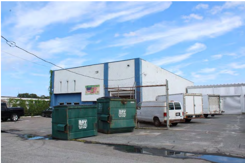
View of building looking northeast
