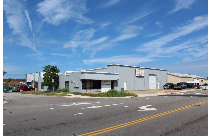
View of building looking northeast
