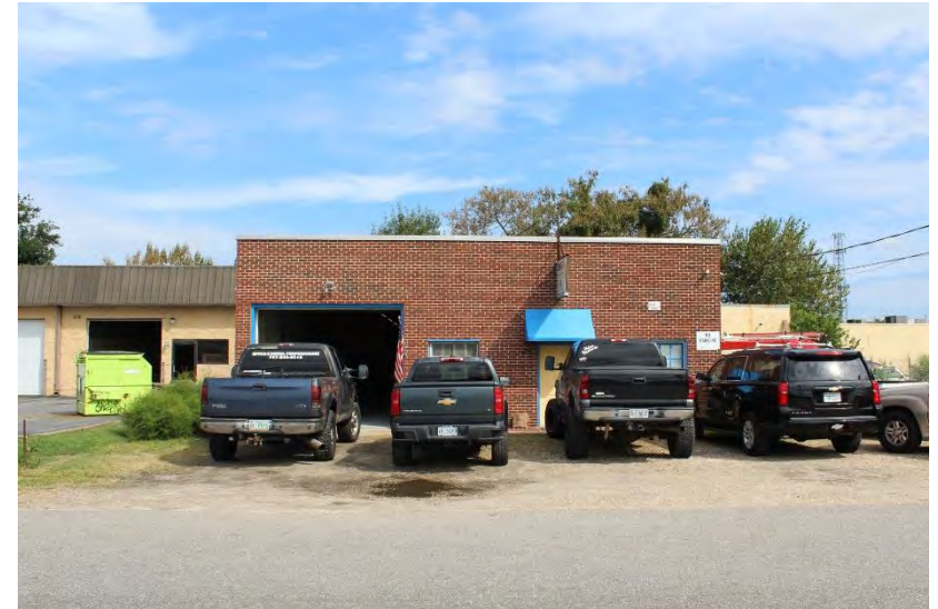
View of building looking east
