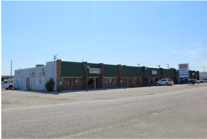
View of building looking southwest
