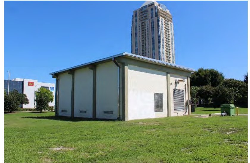
View of building looking northeast
