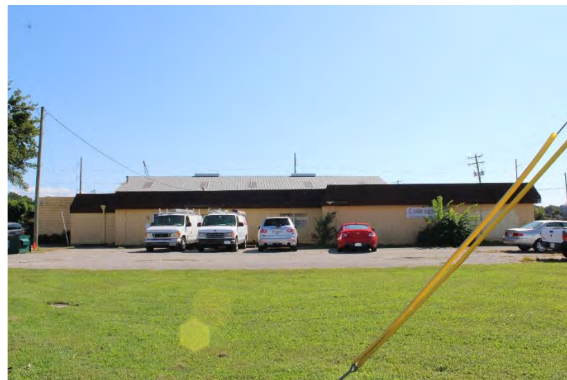
View of building looking south-southwest
