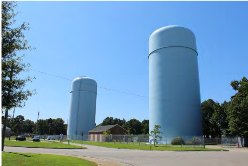
View of water towers and utility building looking southwest
