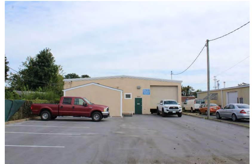
View of building looking east
