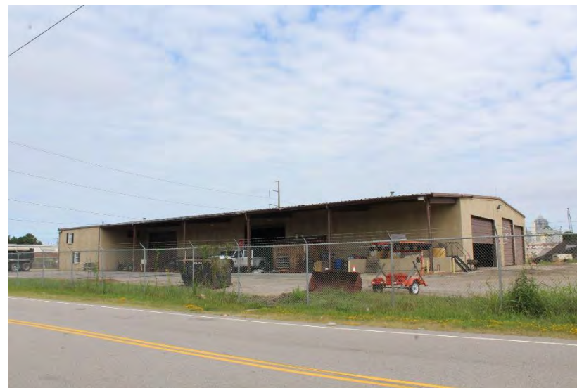
View of building looking northeast
