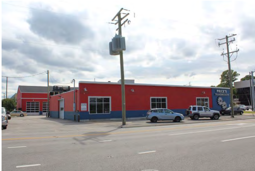
View of building looking southwest
