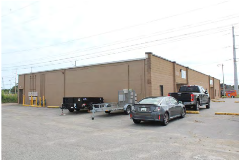
View of building looking south-southeast
