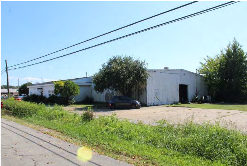
View of warehouse looking south
