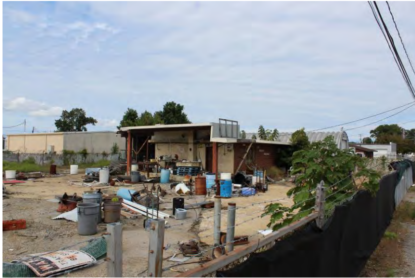
View of building looking northwest
