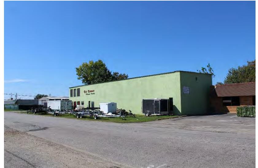
View of building looking northwest
