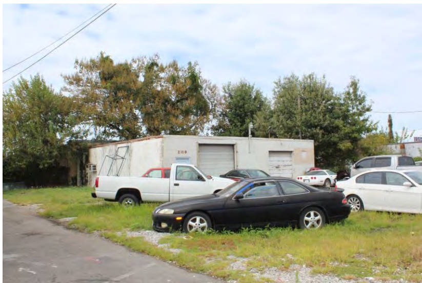
View of building looking northwest
