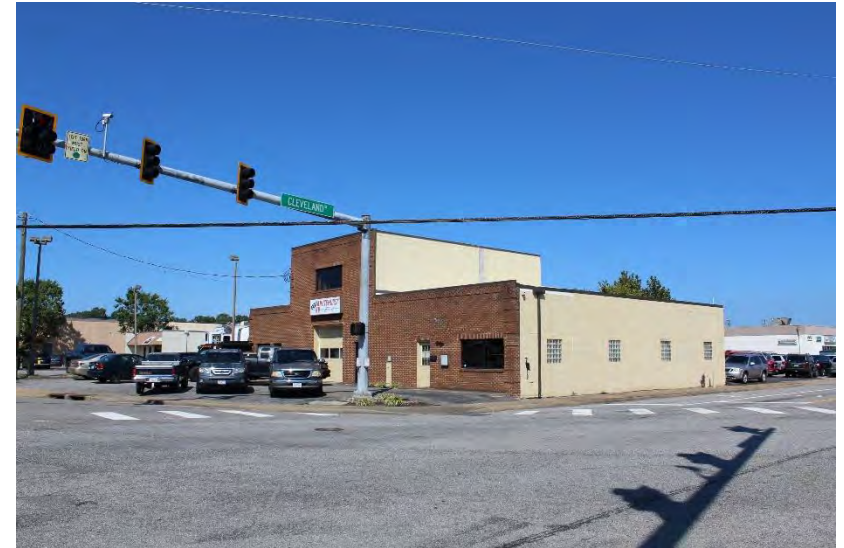
View of building looking northeast
