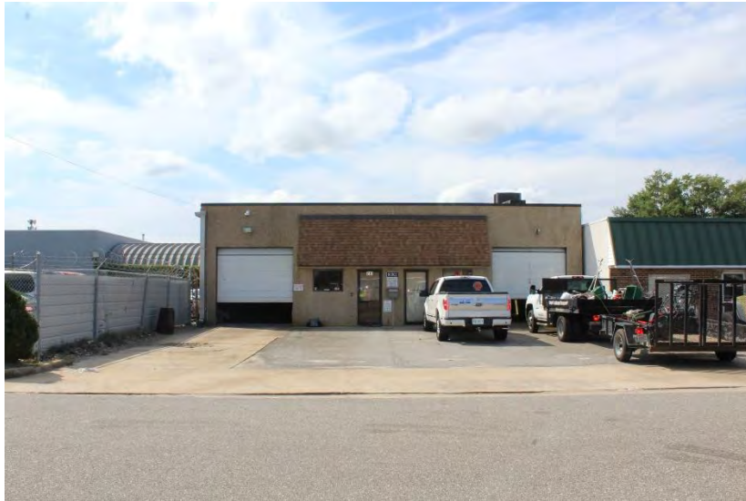
View of building looking west
