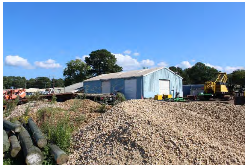
View of Ford Pile Foundation looking southwest
