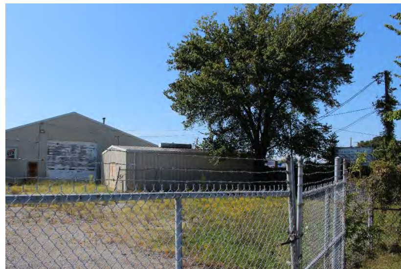
View of building looking northwest
