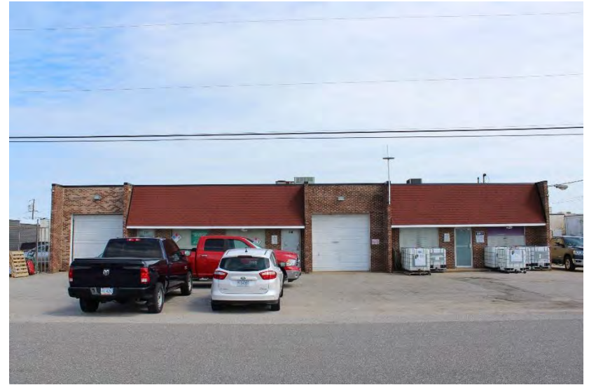
View of building looking east
