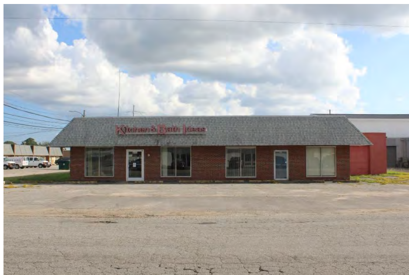
View of building looking south
