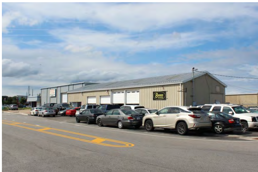
View of building looking northwest
