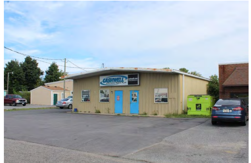
View of building looking northeast
