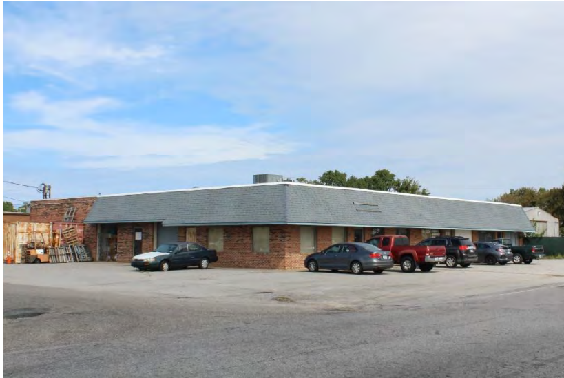
View of building looking northeast
