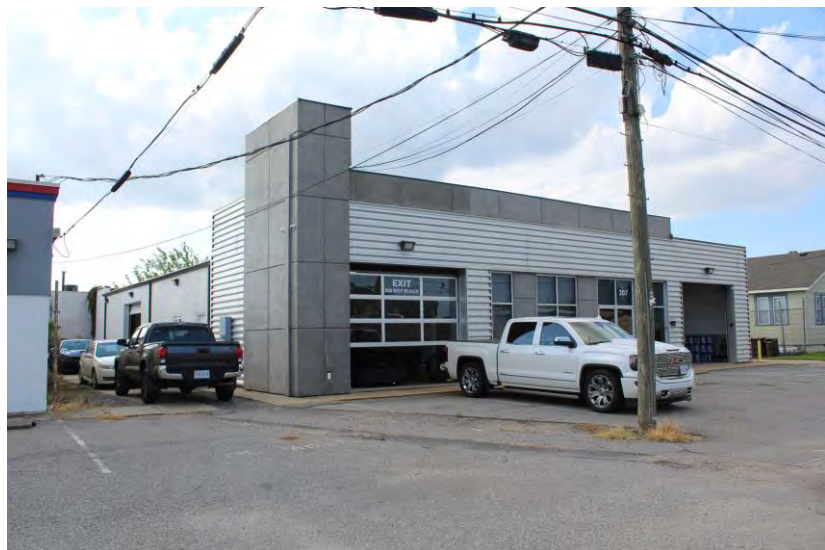
View of garage looking northwest
