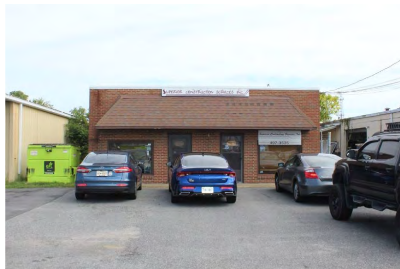
View of building looking east
