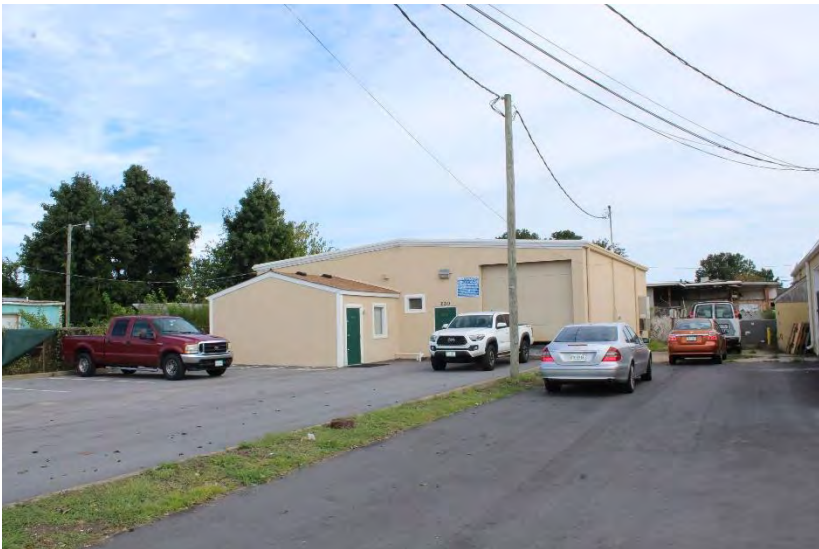
View of building looking northeast
