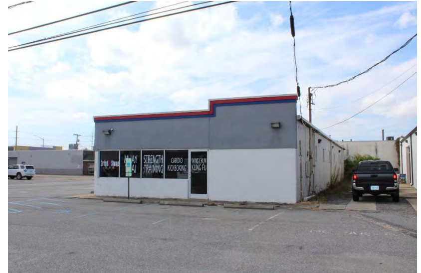
View of building looking southwest
