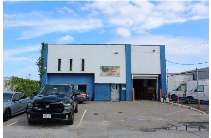
View of building looking east
