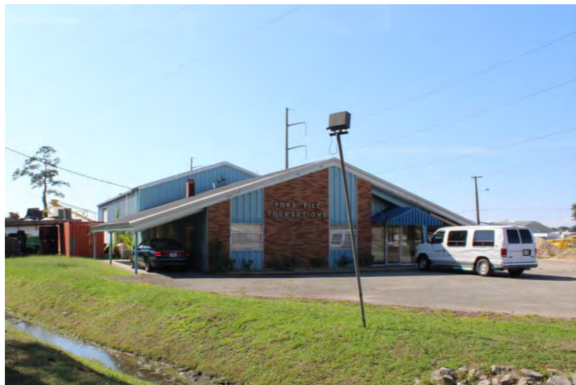
View of Ford Pile Foundation looking northwest
