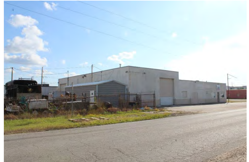
View of building looking southwest
