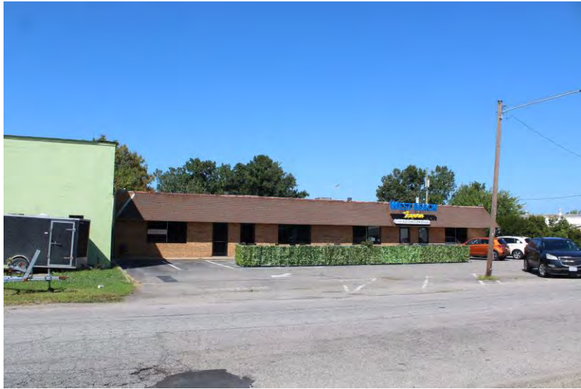
View of building looking northeast
