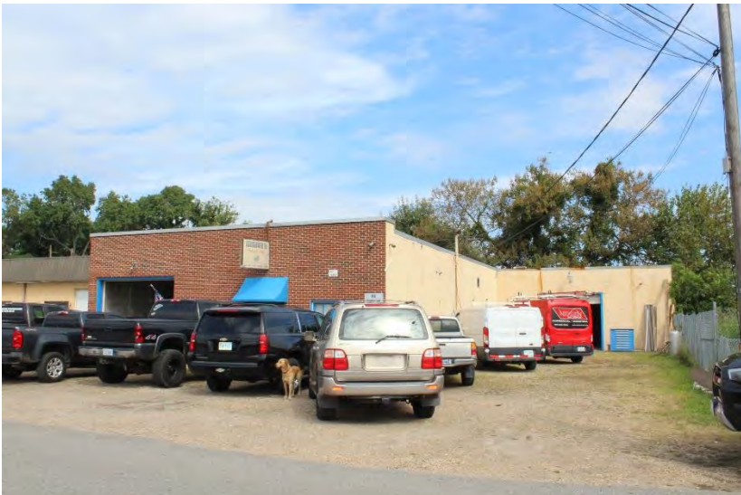
View of building looking northeast
